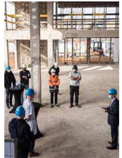
Eerstesteenlegging campus Rumst
