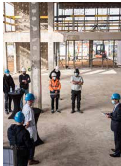
Eerstesteenlegging campus Rumst
